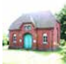
VALVE HOUSE ON VYRNWY -LIVERPOOL AQUEDUCT
