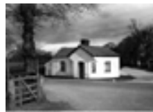
THE FORMER TOLL HOUSE AT HAMPTON
